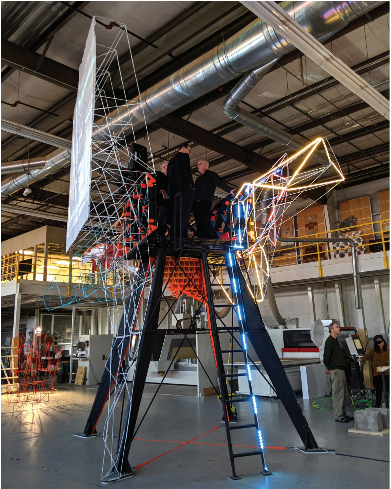
Figure 2. Final installation of Beacon Armature , with spatial frame components designed, fabricated, assembled and installed through MR-based approaches. Spatial Futures Studio.
